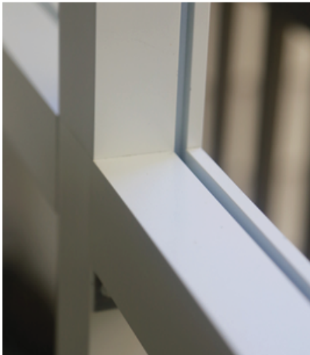
2x2 Chair Rail Installed
